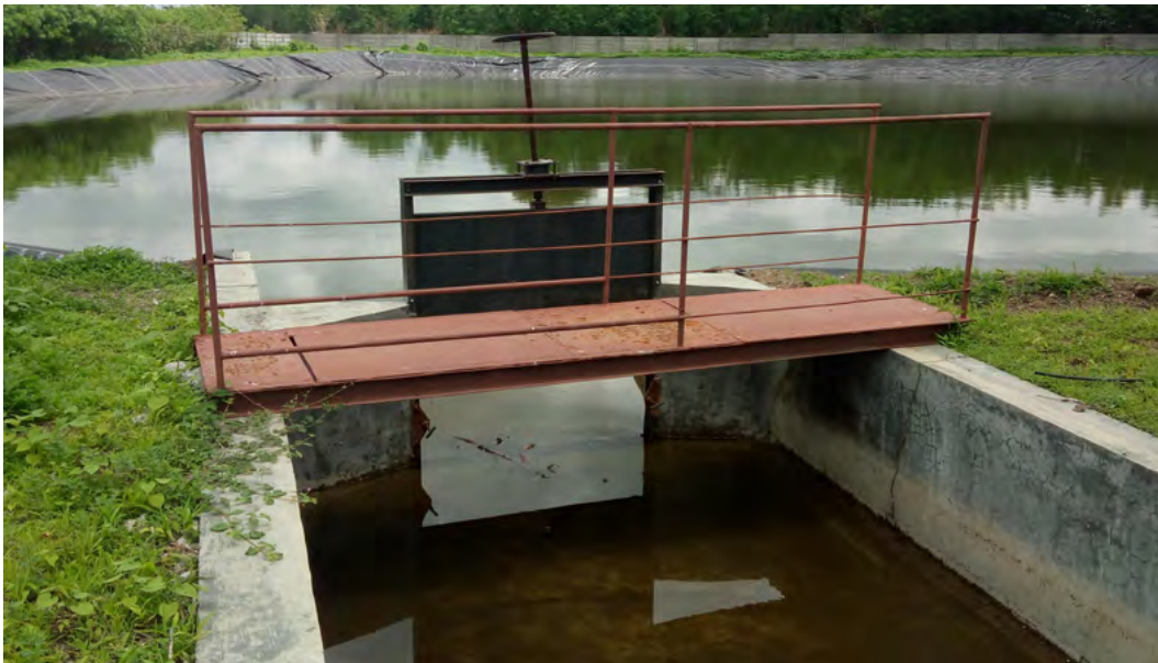
Ground Water Recharge at Waluj
